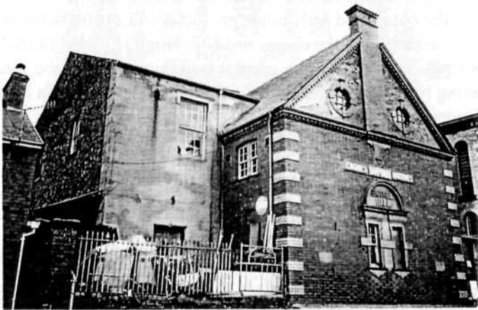
Former Bethel CM Chapel (now ironmonger shop)
