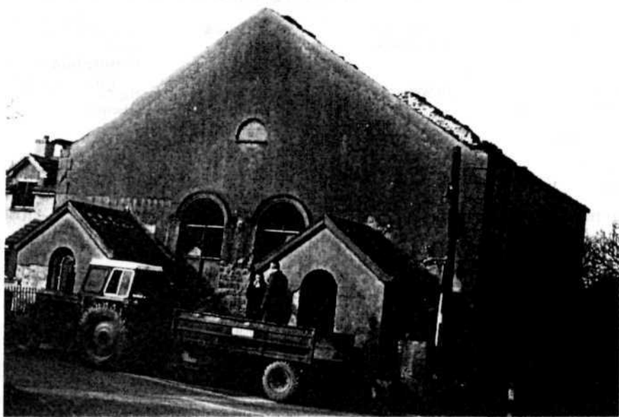
The Presbyterian church at Capel Dewi near Aberystwyth which was closed in 1990, was demolished on the eve of St. David's Day 1993
