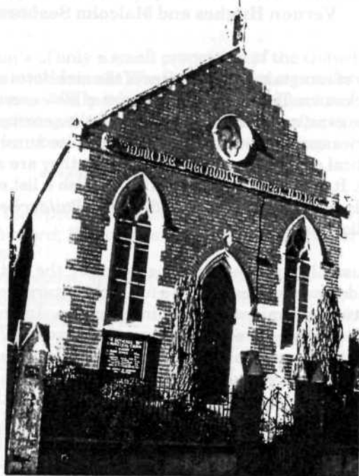
Bethania Evangelical Church Hay on Wye (formerly Oxford Road Primitive Methodist Church)
