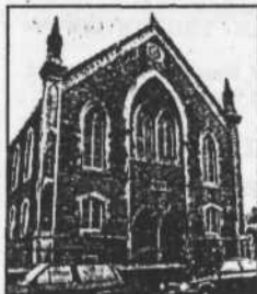
Demolition plans . . . for the Lloyd Street Chapel.
