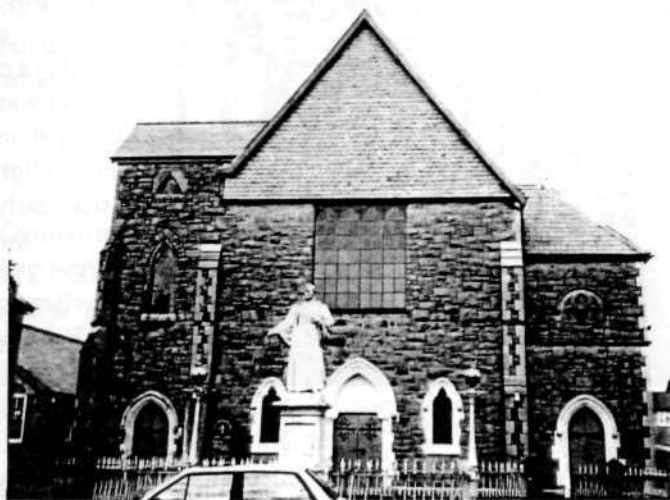
Capel Tegid after demolition of the tower
